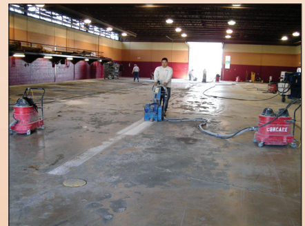
A Concare team member uses a scarifier during the preparation phase.
