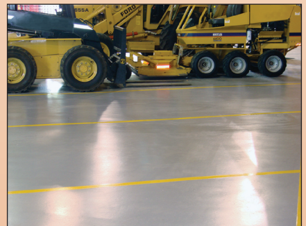
Tough, safe new flooring brought new life to the Alsip Public Works garage.
