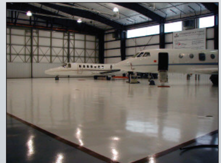
Concare, Inc. provides Elliott Aviation with a beautiful solution to an EPA problem.
