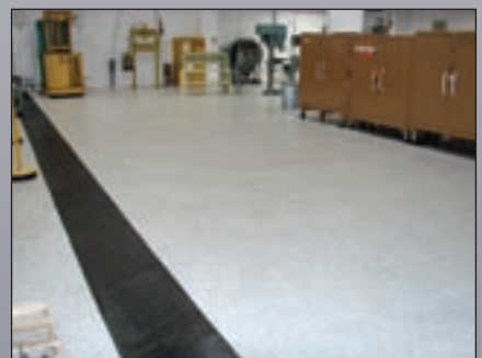
Light reflectivity was increased by 50%, thanks to a new Concare flooring system.
