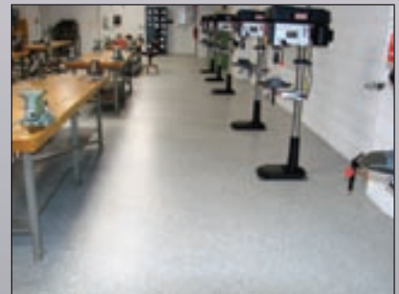
LevelRight MM features an impervious surface that shields concrete below it.
