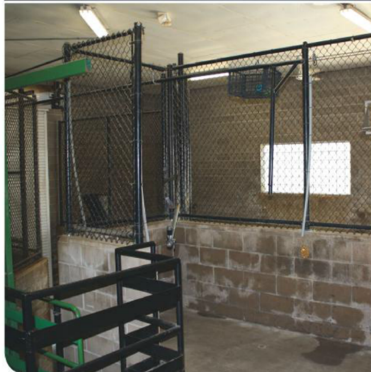
For the 1,715 square-foot (159.3 m 2 ) concrete floor, the six-person Concure crew removed the old mat and mastic and installed a three-layer coating system from Protective Industrial Polymers that included Hoof Guard 36 to act as a natural nail file.
