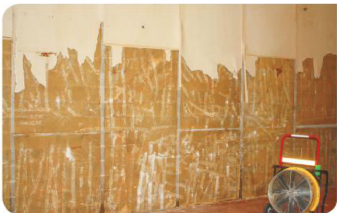
The walls' fiberglass panels (FRP) were deteriorating and needed to be redone. The plan was to use a four-stage coating system, which included a more viscous material than on the floors. But first: prep!
