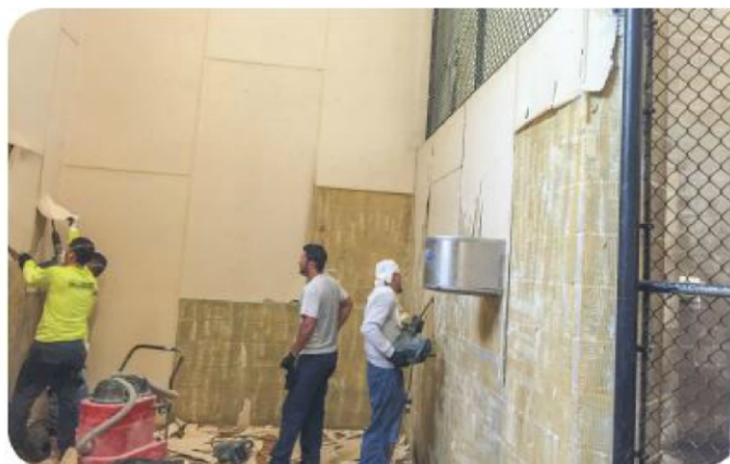
Because of the heights of the enclosures, the crew needed to use scissor lifts at times. They also wore dust masks, safety shoes, safety glasses, and Tyvek protective suits, when necessary.
